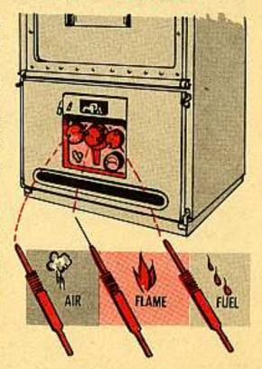
Two of the stems—the air and fuel look alike, except the air stem is a bit shorter. The middle stem—the flame—has a needlepointed end, so you can't mistake it.
