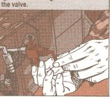
S Use a screwdriver or suitable object small enough to pass through the valve openings to remove the paste-like mess that caused the clog.
